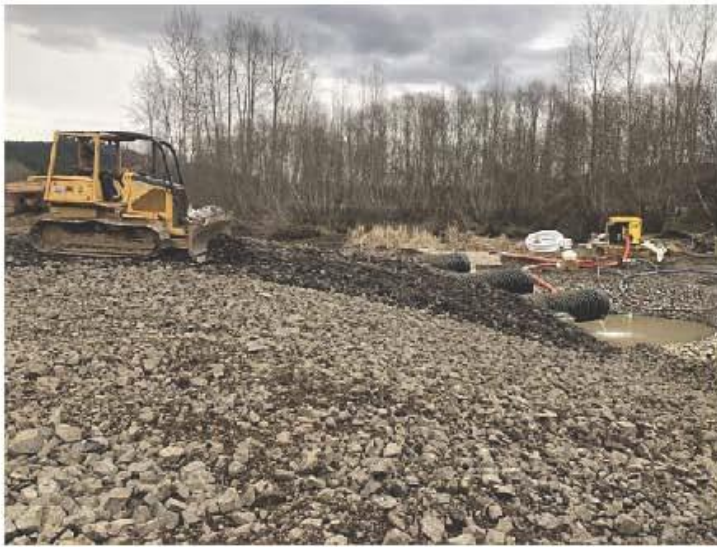
Description: Armoring rock placement
