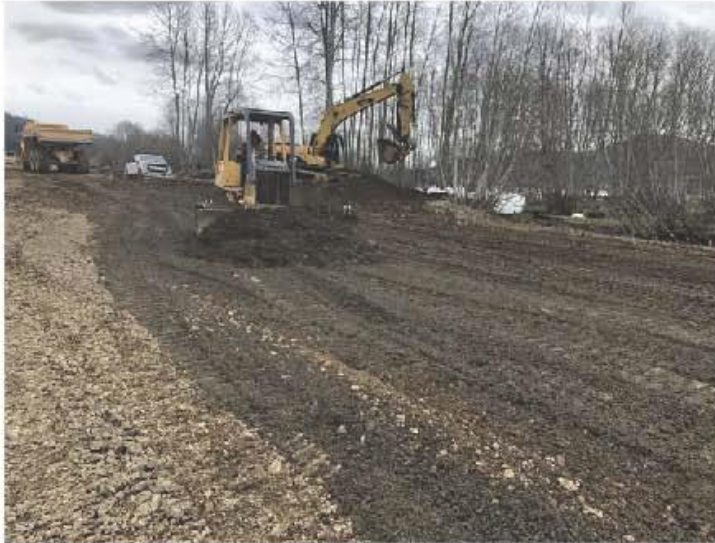
Description: Filter rock placement
