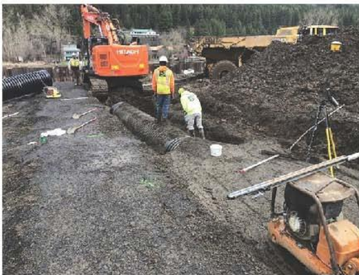
Description: Culvert #4 installation/backfill/compaction
