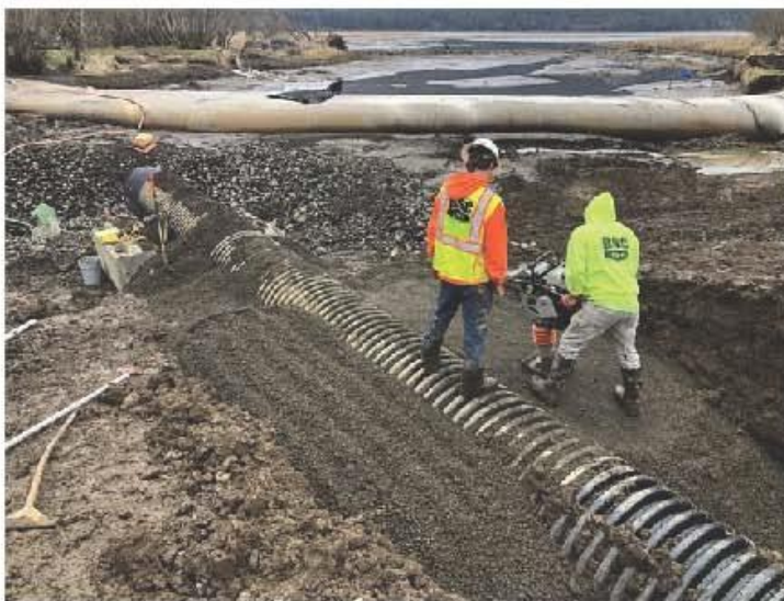
Description: Culvert #1 installation/backfill/compaction
