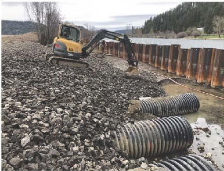
Description: Armoring rock placement at the north toe of slope trench
