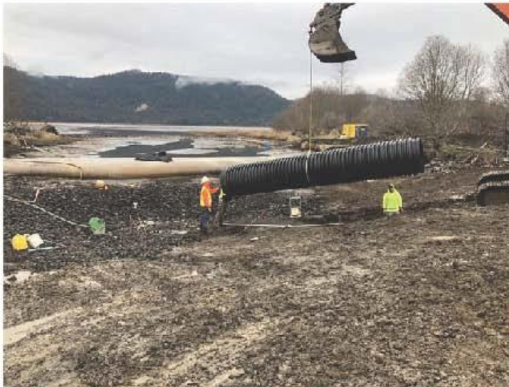
Description: Culvert #1 installation
