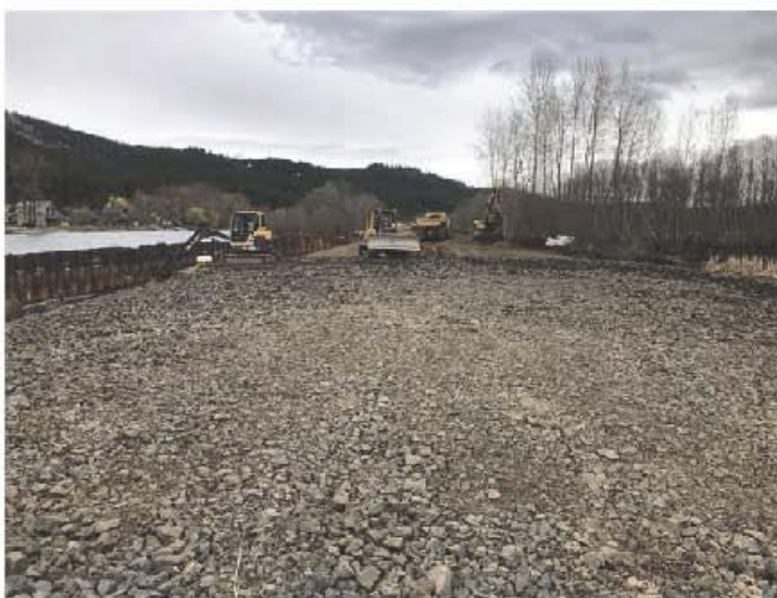
Description: Armoring rock placement
