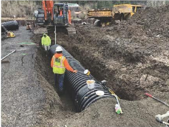
Description: Culvert #4 installation/backfill/compaction
