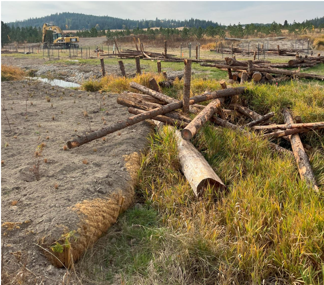
In-channel and floodplain placements of large wood on upper Lake Creek; example of a “floodplain fill cell” is visible (left foreground).
